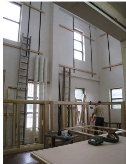
(Case Work being Assembled)
