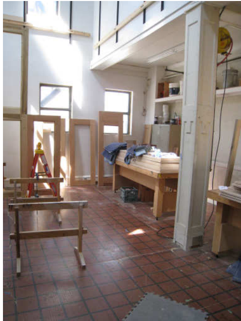
Case Frames and Panels in Assembly Room
