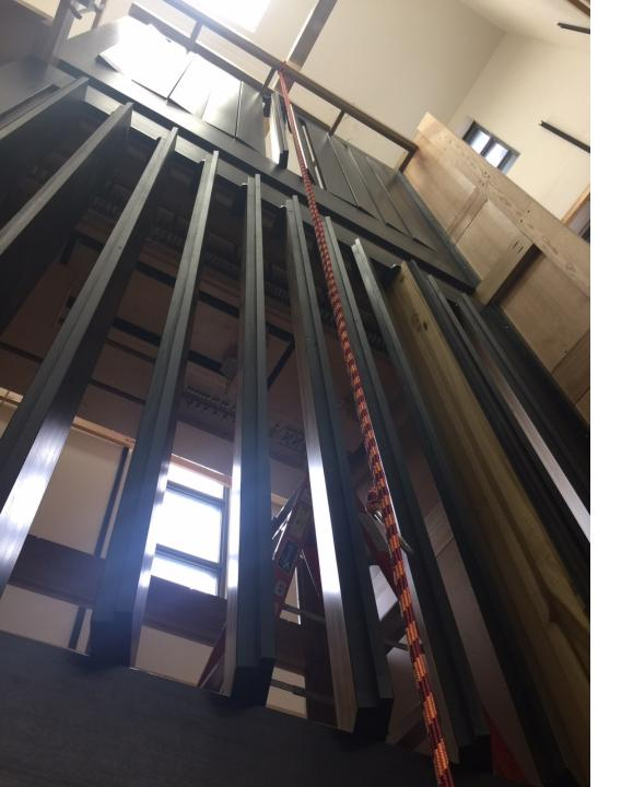
The black wood slats are the swell shades. They will open and shut gradually to create crescendos and diminuendos. They are painted black to be less conspicuous. The façade pipes will be installed in front of the swell shades.
