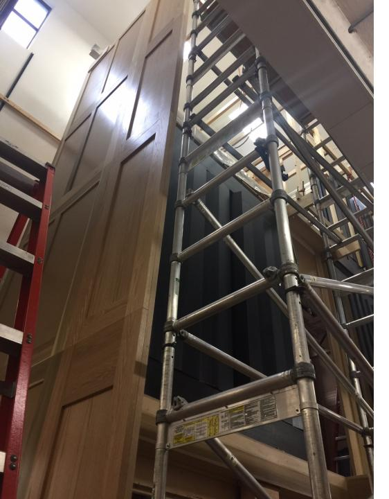
This view shows the side of the red oak case. When the case is built, enough pipes will be installed to test the organ's mechanism. Then it will be disassembled and rebuilt in our sanctuary.
